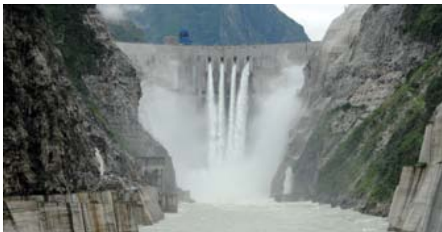
Jinping-1 Project on Yalong River China is the highest arch dam in the world at 305m.
